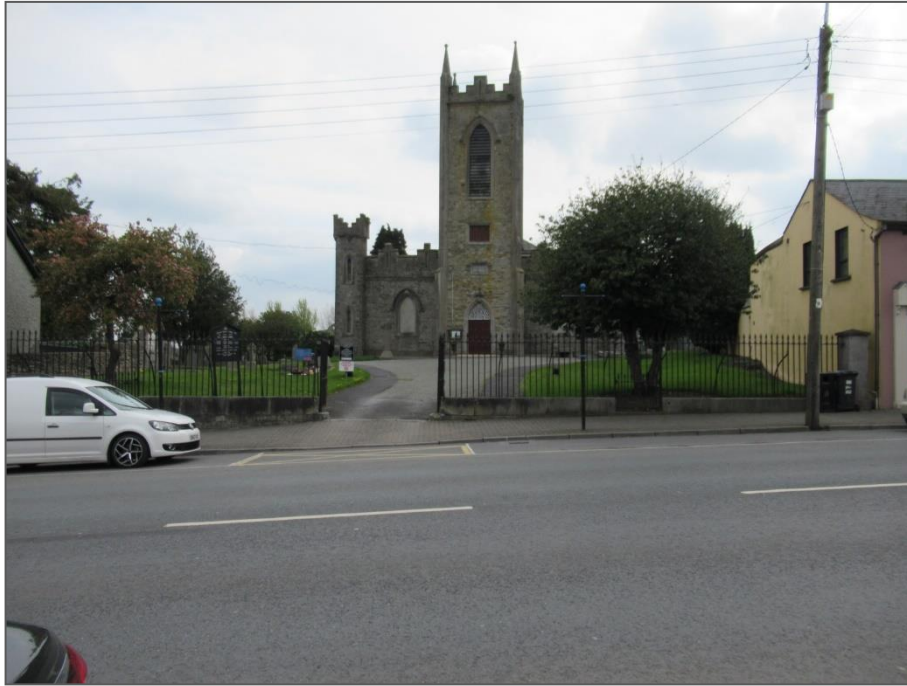
Photo 11: Front elevation of St. Mary's Church, standing within its ancient church yard on the northern end of Main Street. Most of the present structure dates from the C19th, however the remains of a small ancient chapel were incorporated into this structure. The church yard has many beautiful old and ancient gravestones.
