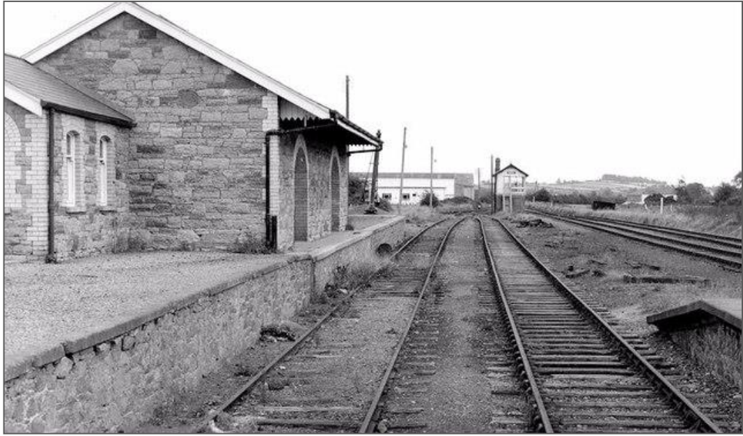
Photo 19: Historic photo showing the original Goods Shed on the raised platform. That structure was removed after the station was closed during the late C20th.
