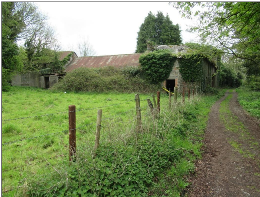
Photo 14: View looking south, from the same location as the previous photo, showing the historic farmyard previously associated with Ardee House. At the right side of the yard, at the rear, is another late medieval tower house, originally standing outside of the protective walls of Ardee.
