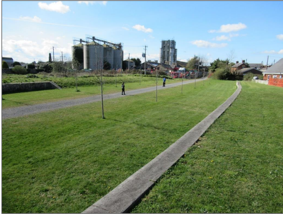
Photo 15: General view looking west across the Railway Lands area. The Victorian station and adjacent engine house are visible in the distance, now in separate commercial use. The raised passenger platform is visible at left.
