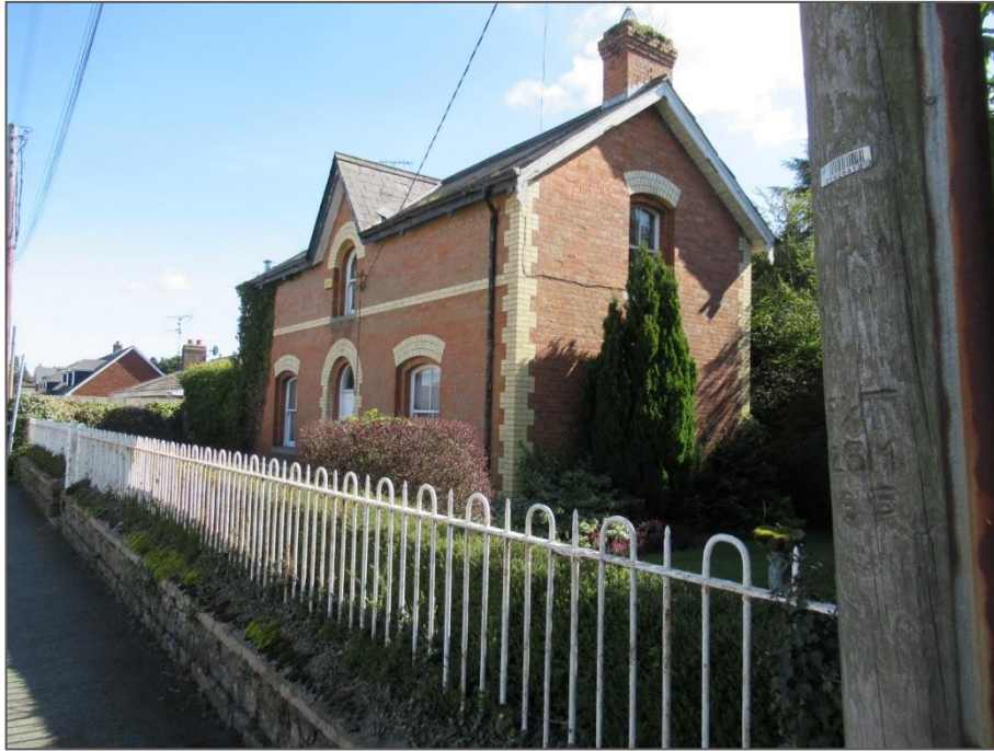
Photo 21: General view showing the front elevation of the former Station Master's House, Sean O'Carroll Street. This fine house is now in private use but remains unchanged from its original appearance.
