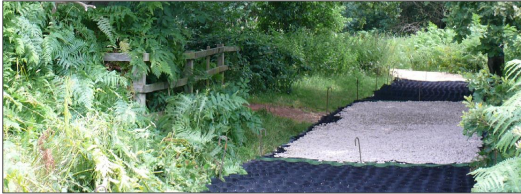
Figure 5.6: The Installation of a Cellular Confinement System
