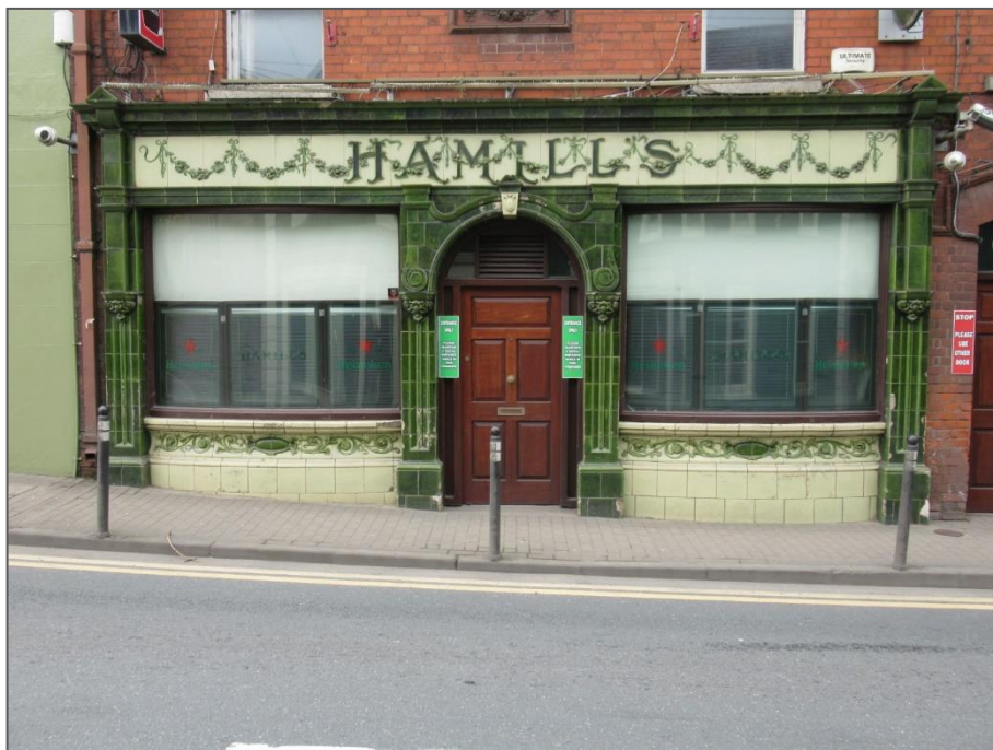
Photo 9: Excellent terra cotta shop front on a historic pub, located on the west side of Bridge Street, on the south bank of the River Dee.
