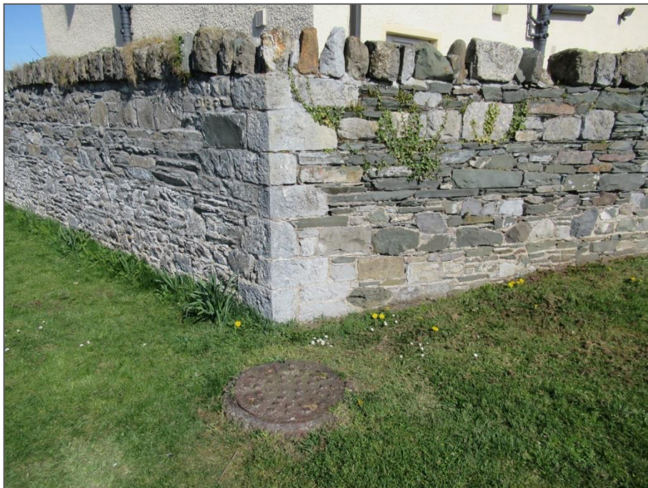
Photo 18: Detail view showing the fine limestone rubble masonry wall that survives from the railway station area.
