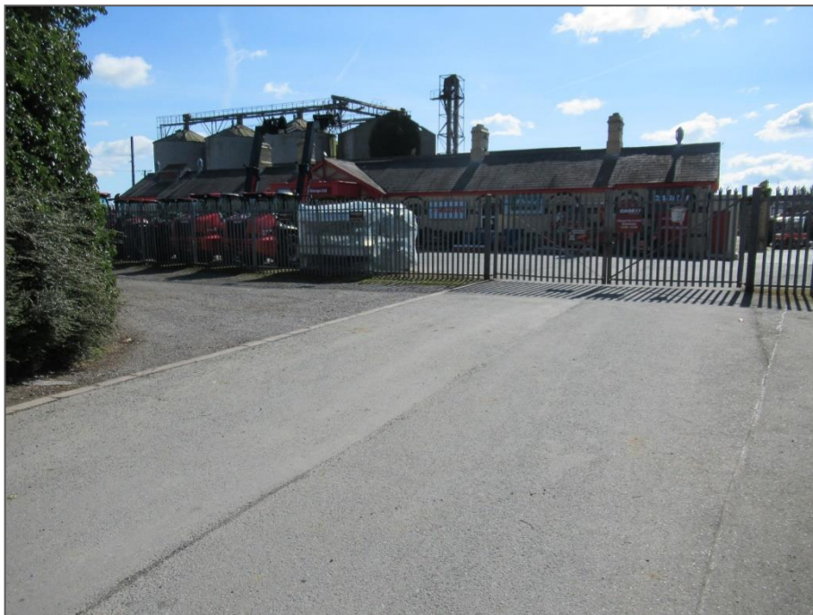
Photo 16: General view looking south showing the former station, currently in use as a heavy plant dealership.
