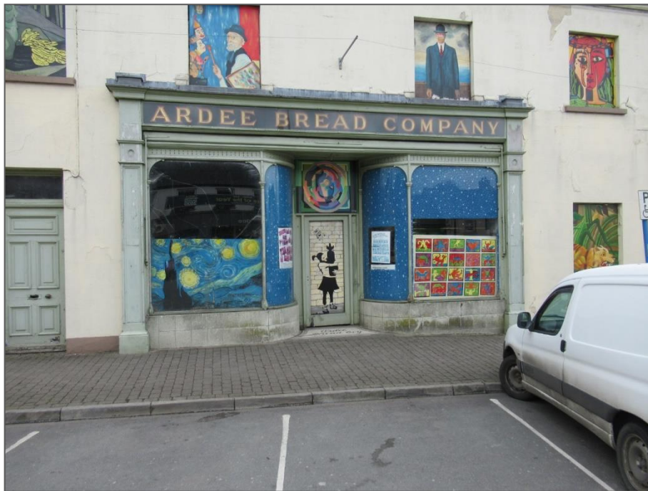
Photo 8: Victorian period shop front on a disused shop on the east side of Main Street.
