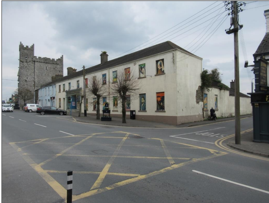
Photo 4: Recent photo looking north along the east side of Main Street, showing the castle at left, flanked by a terrace of largely empty and underused historic structure.
